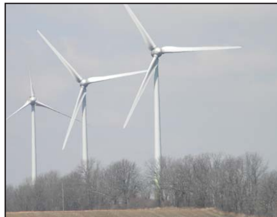
There are 43 wind turbines on the property, each measuring 80m (260') in height with each blade reaching 47.55m (156') in length.
